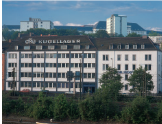
Administration and production facilities in Würzburg
